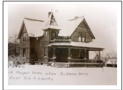
Arnoldus and Marie Kuyper's home. Built in 1890 – 614 E. 3 rd . Street Pella. It was here they raised their 3 boys, Peter, Lou and Bob.
