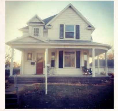
The home of Lee & Juli White after renovation (top) & showing its potential (bottom)
