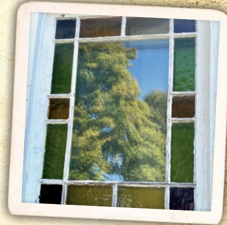
An example of a Pella window "rimmed with small, varicolored panes of glass"
